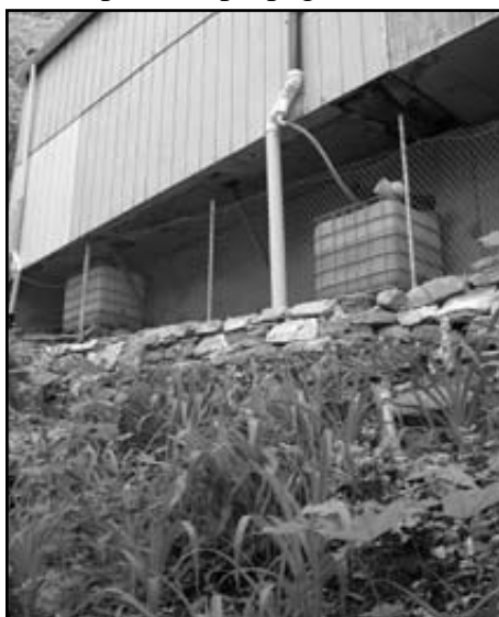
Irrigation system installed. Native species now replace the non-native iris and daffodils holding riverbank in this photo.
