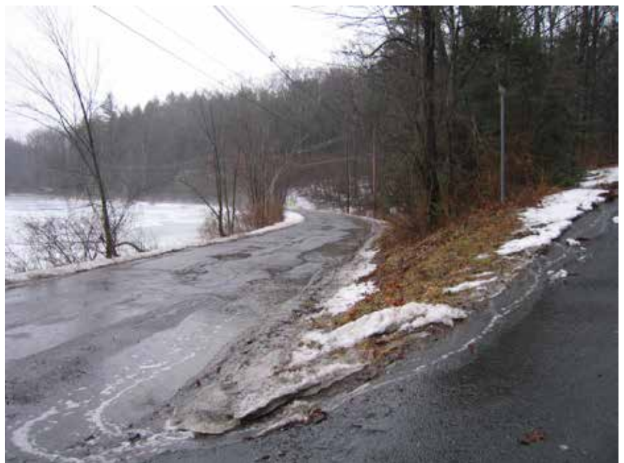
Rainwater and snowmelt from Knob Hill Road
